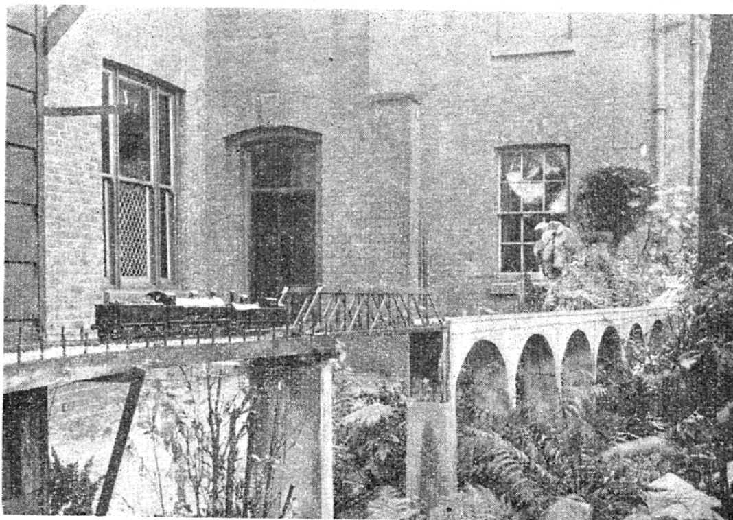
Fig. 2. View on the single-line portion, showing pre-cast concrete viaduct and hinged girder bridge
