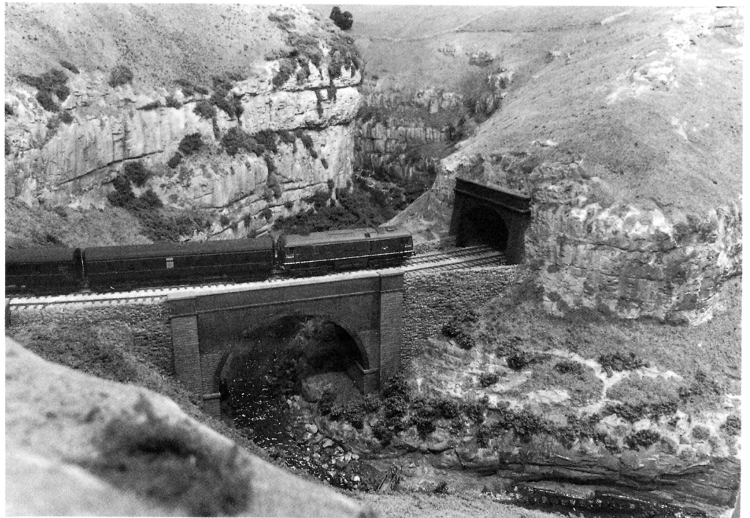
BR/Sulzer Type 2 diesel crossing Chee Tor Bridge with a Buxton-Derby semi-fast train which is about to enter Chee Tor No. 1 Tunnel. This double track bore was driven through a short limestone spur. The limestone cliff face of Chee Tor rises up behind the bridge.
