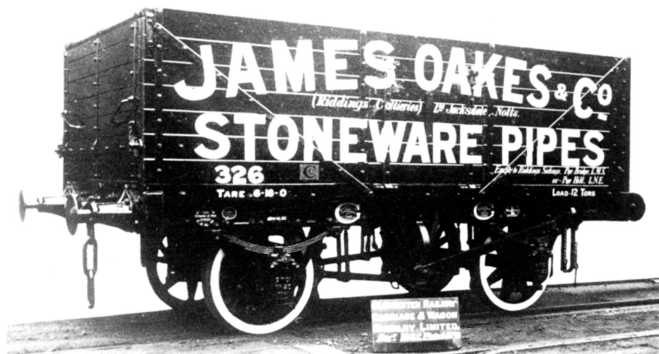
Not a stoneware pipe wagon, but a coal wagon. It is secondhand, and would originally have run in South Wales (toothed brake rack, commode handles, foot-treads on buffers). James Oakes & Co. were colliery owners. The wagon is to 1907 specification. GRC & W Co.
